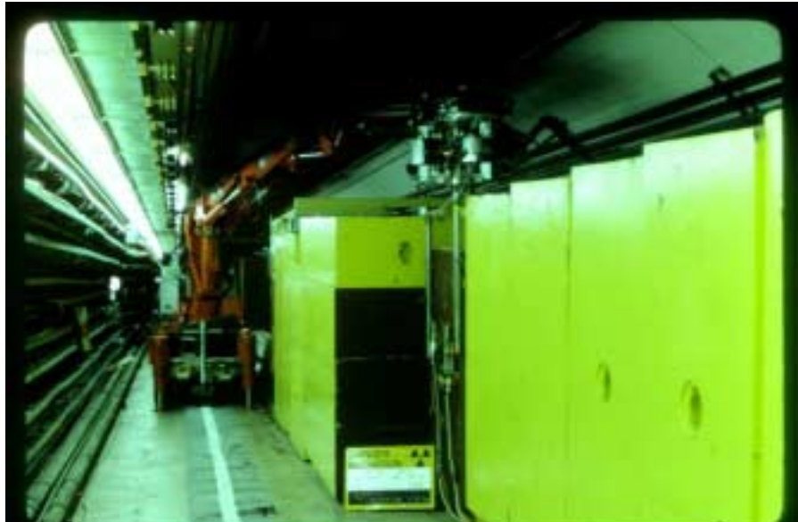
In the Tunnel
