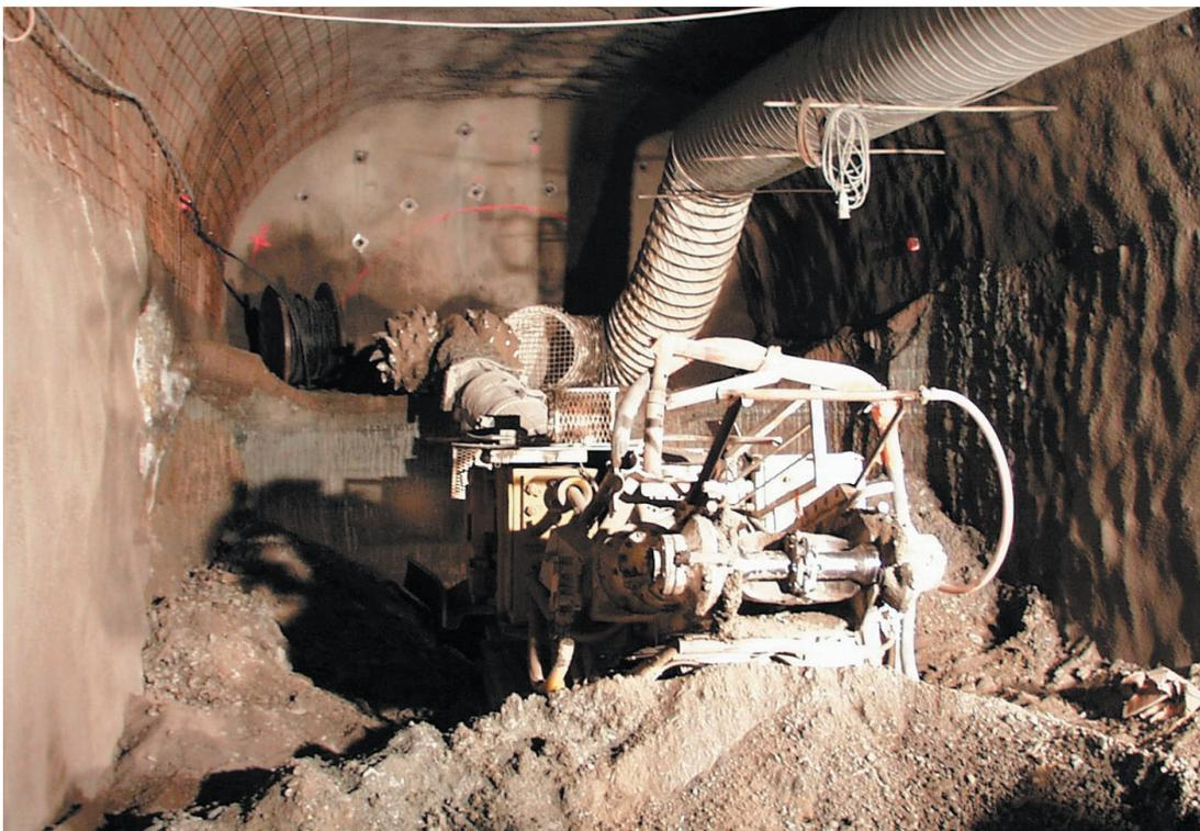
**Figure 15:** Excavation with rotating head boring machine (roadheader)
