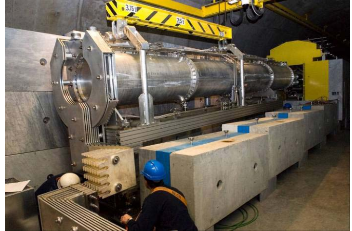
Fig. 6. The CNGS horn during installation.
