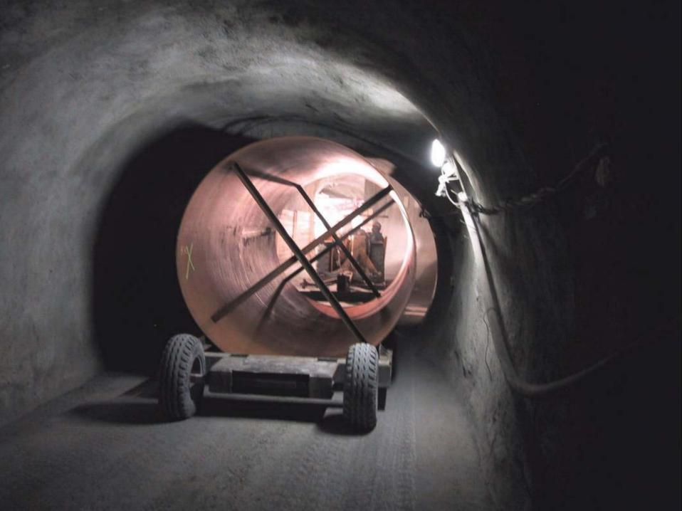
target chamber: assembling the 18m long section
