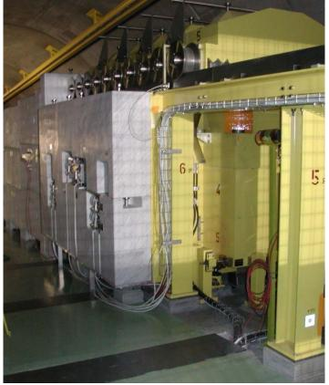
• Remote exchange of radioactive items like target, horn, reflector and collimators in case of a failure. The crane console is located in the ventilation chamber... camera is mounted on crane.
