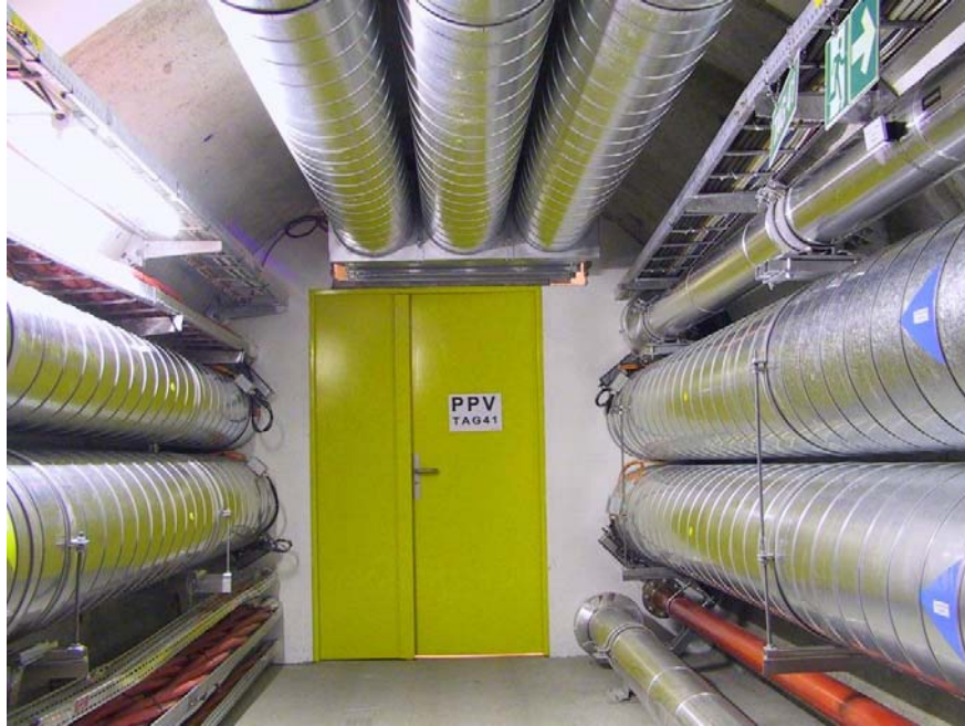
Figure 14: Door PPV TAG41, seen from the access point in ECA4
